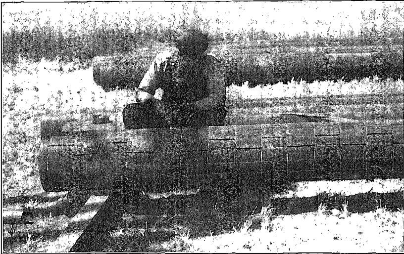
FIG. 61. Perforating 14-in. well casing with acetylene torch. The sections of casing are welded together as they are put into the well. (U.S.D.A. Circ. 546.)
