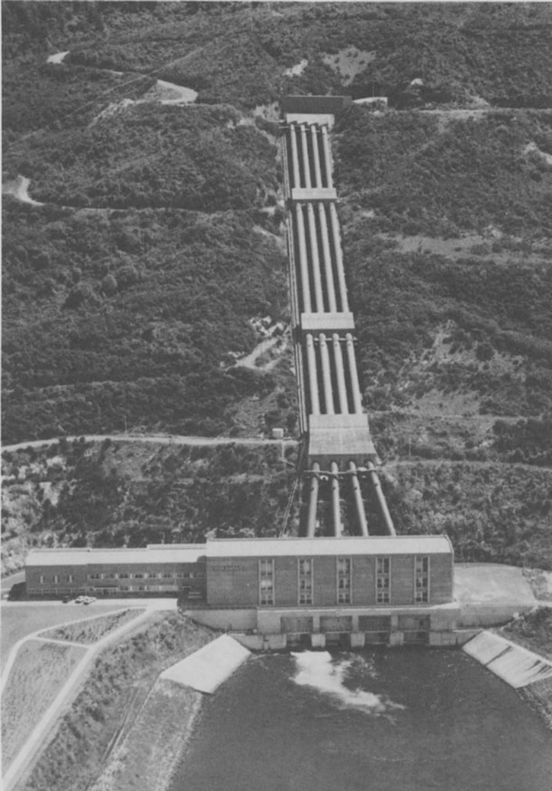
Figure 9.8 Tongariro Hydroelectric Power Station, New Zealand (source: Sir Alexander Gibb & Partners)
