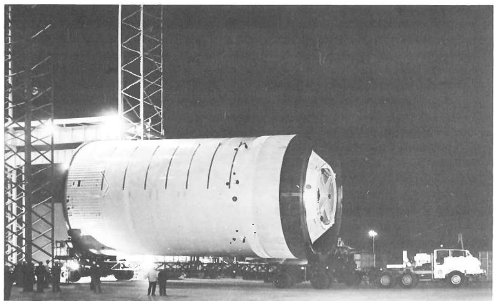
S-11 Hydrogen-fueled booster vehicle, the 81.5-foot tall second stage of NASA's Saturn V Apollo Moon Rocket, was assembled vertically in tower ( top left ) at Huntsville, Alabama; it is seen in turnover station ( top right ) and aboard truck that took it to Cape Kennedy where it was installed atop the giant Saturn V. It is thought to be the most powerful hydrogen-fuel booster in any nation's space program.
