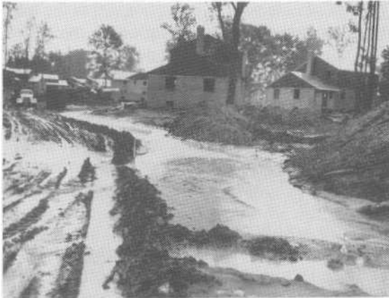
FIGURE 7.1 Removal of the vegetative cover increases water runoff and leaves soil unprotected from the erosive effects of the rain, resulting in accelerated soil erosion. As water concentrates in channels, its erosive power increases. (Photograph courtesy Soil Conservation Service, USDA.)
