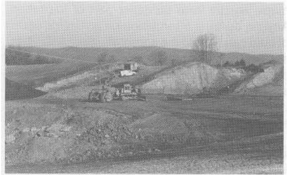
FIGURE 19.5 Sites selected for solid waste disposal (landfills) need water-impermeable underlying strata to minimize groundwater pollution.
