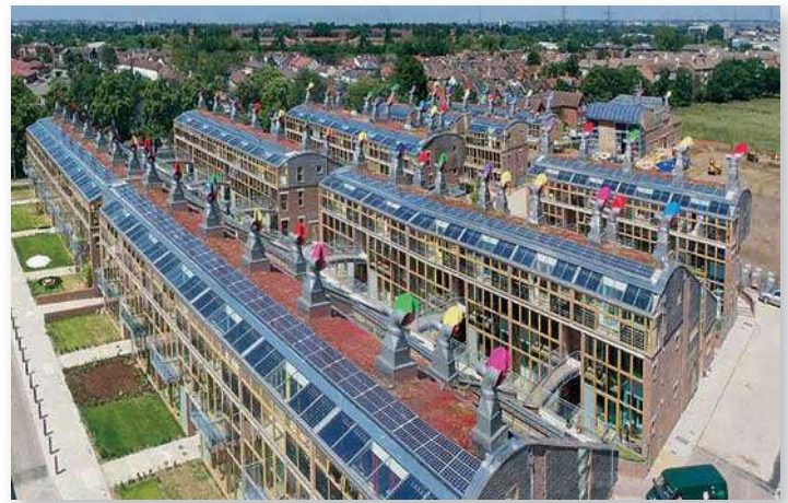
South-facing windows heat homes, and colorful, rotating "wind cowls" ventilate rooms at BedZED, an ecological housing complex in South London, U.K.
