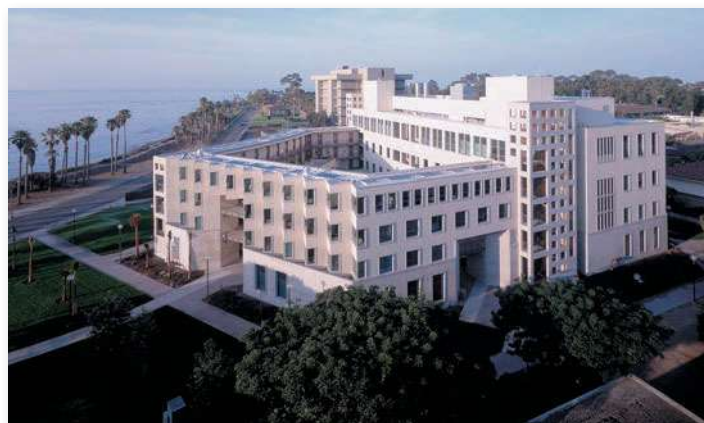
FIGURE 25.13 The University of California at Santa Barbara claims its new Bren School of Environmental Science and Management is the most environmentally friendly building of its kind in the United States.
