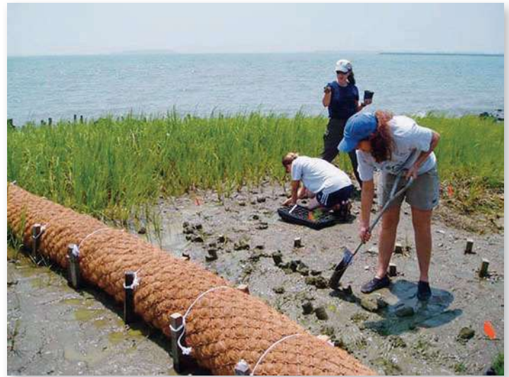
FIGURE 13.27 Volunteers plant dune grasses as part of Chesapeake Bay restoration. Ultimately, this effort hopes to revegetate at least 200,000 ha of coastline, salt marsh, and shallow water areas of the bay. The large cylinder is a "bio log" made of biodegradable material that will help stabilize the shore. Source: NOAA.
