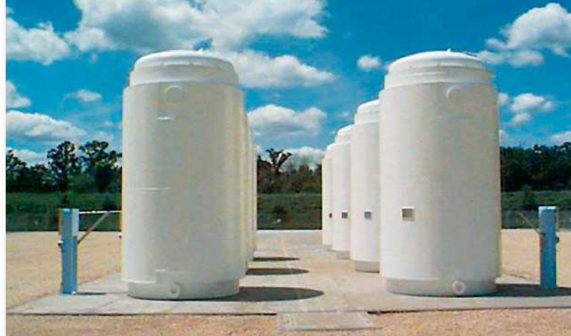
FIGURE 19.25 Spent fuel is being stored temporarily in large, aboveground “dry casks” at many nuclear power plants.
