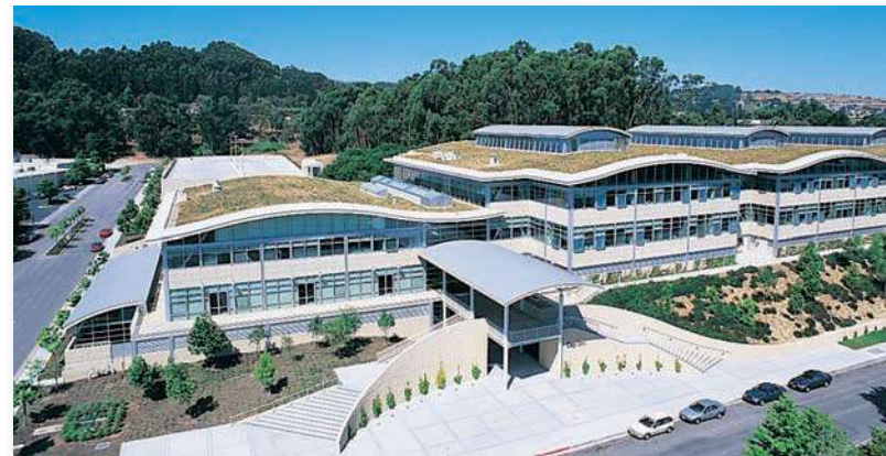
FIGURE 23.25 The award-winning Gap, Inc. corporate offices in San Bruno, California, demonstrate some of the best features of environmental design. A roof covered with native grasses provides insulation and reduces runoff. Natural lighting, an open design, and careful relation to its surroundings all make this a good place to work.
