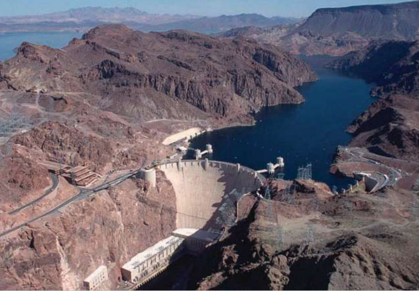
FIGURE 17.22 Hoover Dam powers Las Vegas, Nevada. Lake Mead, behind the dam, loses about 1.3 billion m 3 per year to evaporation.
