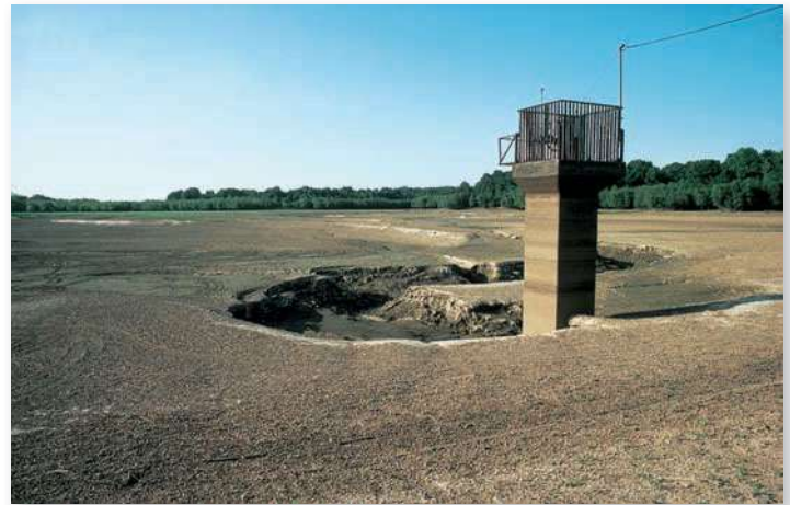
FIGURE 17.23 This dam is now useless because its reservoir has filled with silt and sediment.
