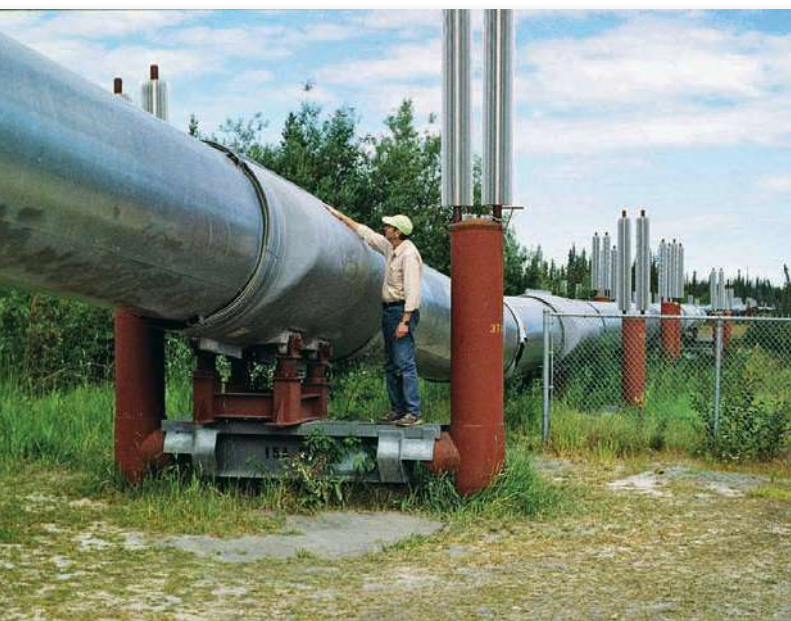
FIGURE 19.14 The Trans-Alaska pipeline snakes for more than 800 miles across Alaska's mountains and tundra. It has been damaged numerous times both accidentally and by vandals. Now melting permafrost and corrosion threaten more oil spills.
