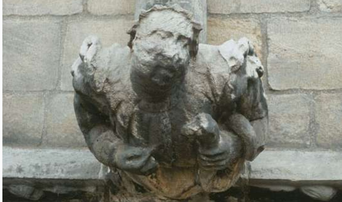
FIGURE 16.28 Atmospheric acids, especially sulfuric and nitric acids, have almost completely eaten away the face of this medieval statue. Each year, the total losses from air pollution damage to buildings and materials amounts to billions of dollars.
