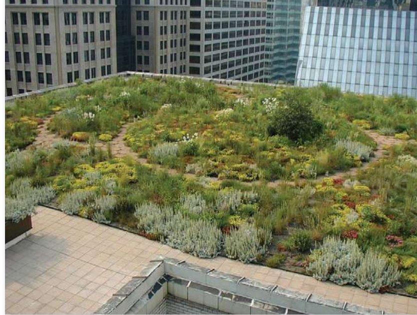
FIGURE 22.20 This award-winning green roof on the Chicago City Hall is functional as well as beautiful. It reduces rain runoff by about 50 percent, and keeps the surface as much as 30°F cooler than a conventional roof on hot summer days.
