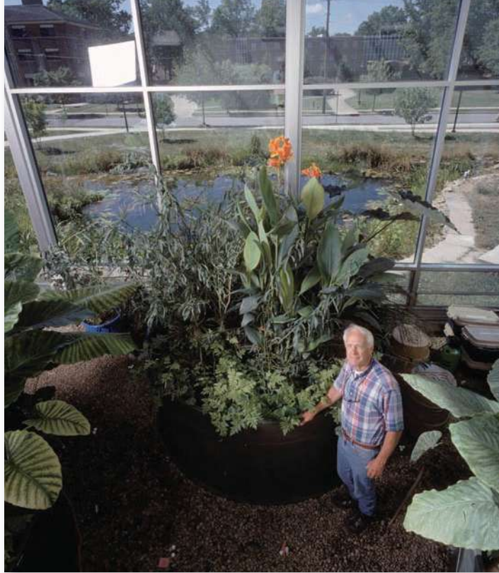
FIGURE 18.27 In-house wastewater treatment in Oberlin College's Environmental Studies building. Constructed wetlands outside, and tanks inside, allow water plants to filter water and use nutrients.
