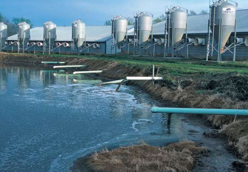
FIGURE 9.14 This state-of-the-art lagoon is built to store manure from a hog farm. Odors and overflow after storms are risks of open lagoons, but more thorough waste treatment is expensive.
