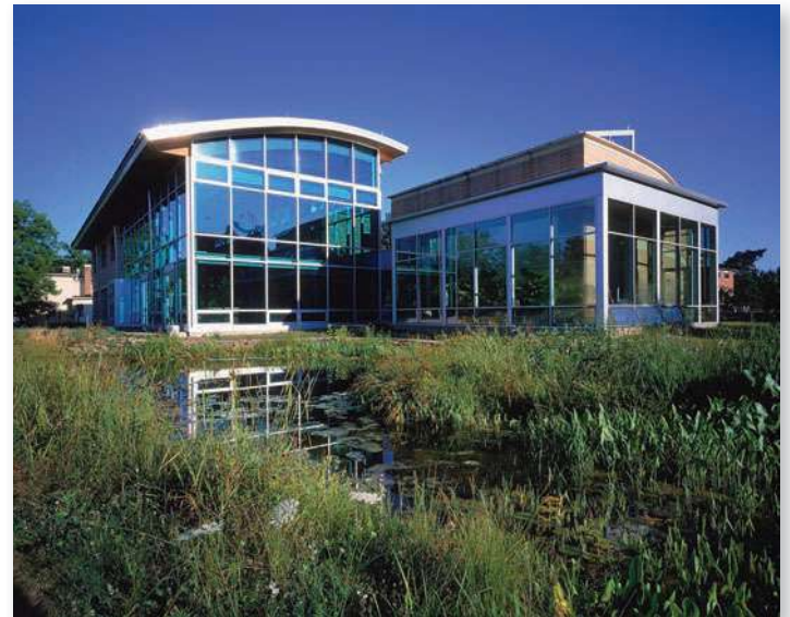
FIGURE 20.9 The Adam Joseph Lewis Center for Environmental Studies at Oberlin College is designed to be self-sustaining even in northern Ohio’s cool, cloudy climate. Large, south-facing windows let in sunlight, while 370 m 2 of solar panels on the roof generate electricity. A constructed wetland outside and a living machine inside (see fig. 18.27) purify wastewater.
