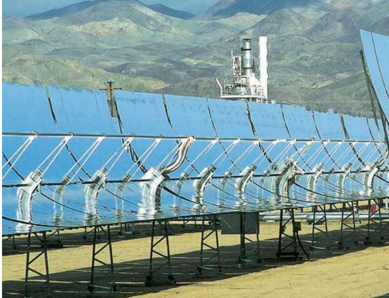
FIGURE 20.10 Parabolic mirrors focus sunlight on steam-generating tubes at this power plant in the California desert.
