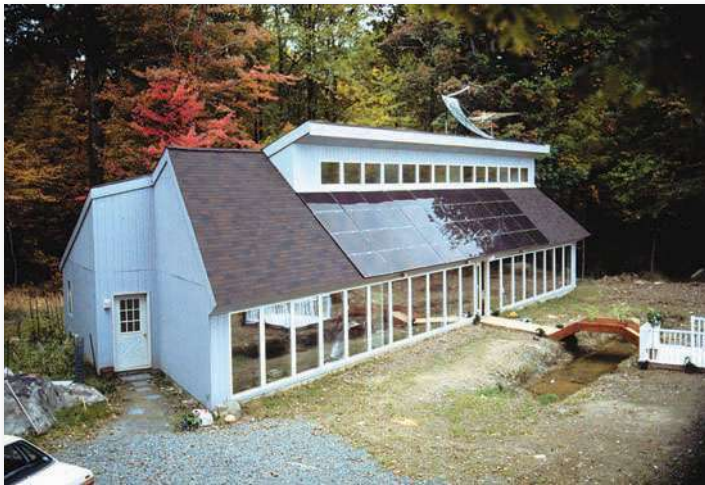
FIGURE 20.13 Roof-mounted solar panels (shiny area) can generate enough electricity for a house full of efficient appliances. On sunny days, this array can produce a surplus to sell back to the utility company, making it even more cost efficient.
