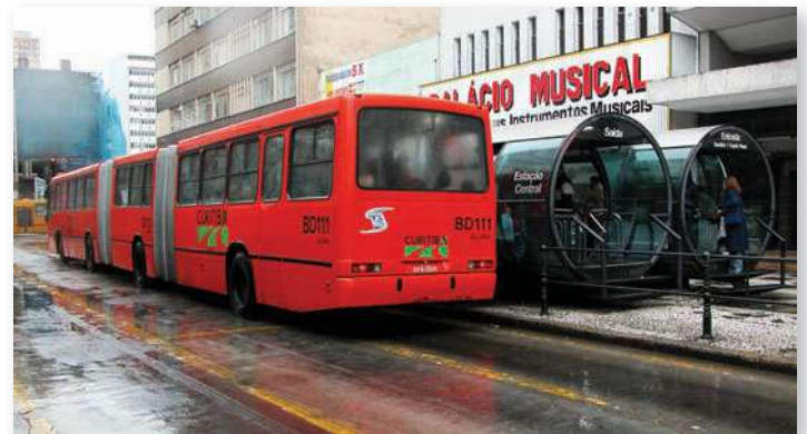
FIGURE 22.17 High-speed, bi-articulated buses travel on dedicated transit ways in Curitiba and make limited stops at elevated tubular bus terminals that allow many passengers to disembark and reload during 60-second stops.
