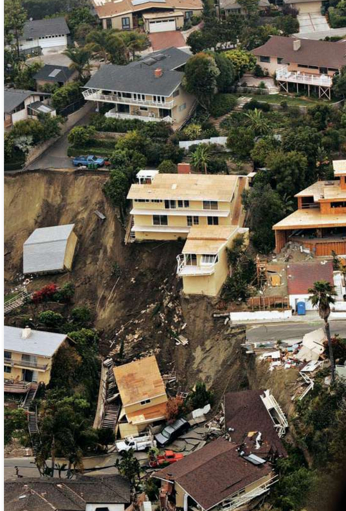
FIGURE 14.21 Damaged homes sit on a hillside after a landslide in Laguna Beach, Calif.
