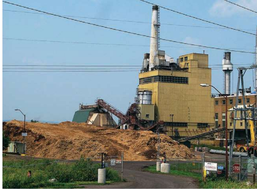
FIGURE 20.19 This Michigan power plant uses wood chips to fuel its boilers. Where wood supplies are nearby, this is a good choice both economically and environmentally.
