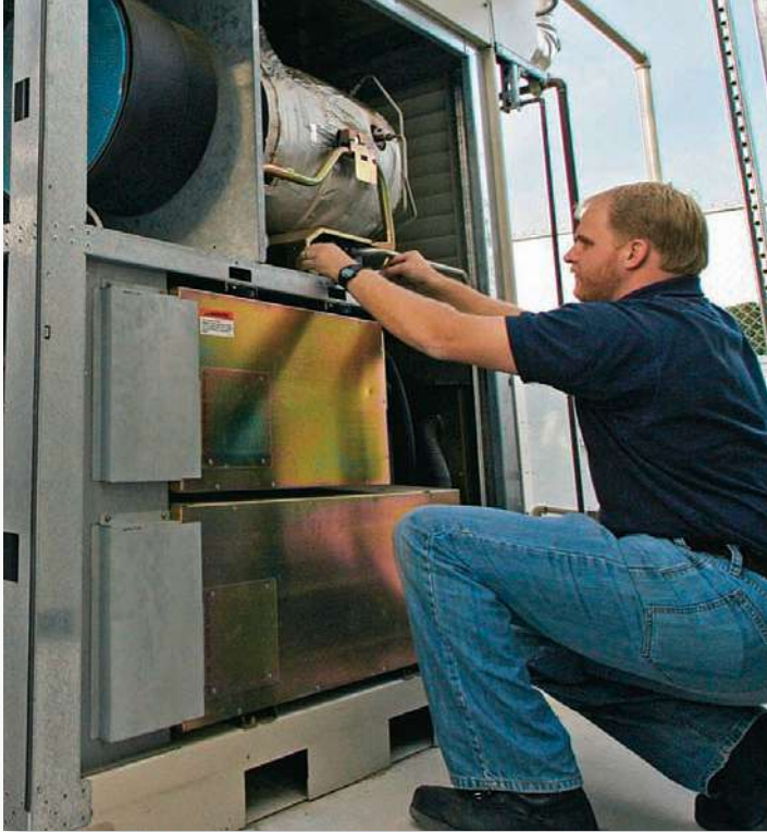
FIGURE 20.6 A technician adjusts a gas microturbine that produces on-site heat and electricity for businesses, industry, or multiple housing units.
