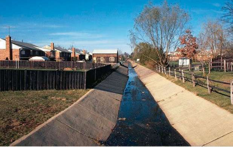
FIGURE 13.30 Many former streams have been turned into concrete-lined ditches to control erosion and speed runoff. The result is an artificial system with little resemblance to the living biological community that once made up the stream.
