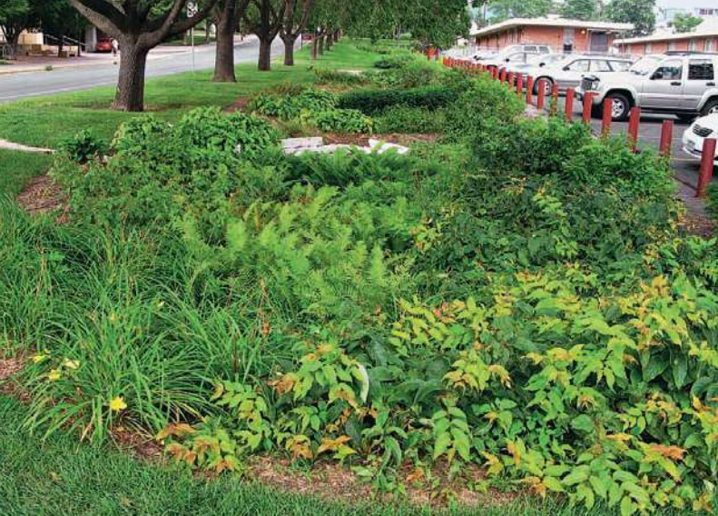
FIGURE 18.28 A rain garden is a shallow depression situated to collect runoff from streets or parking lots. It's planted with species that can survive in saturated soils. This vegetation helps evaporate and cleanse runoff, while temporary storage in the basin allows groundwater recharge. You might build a rain garden in your yard, or on your campus, or elsewhere in your city.
