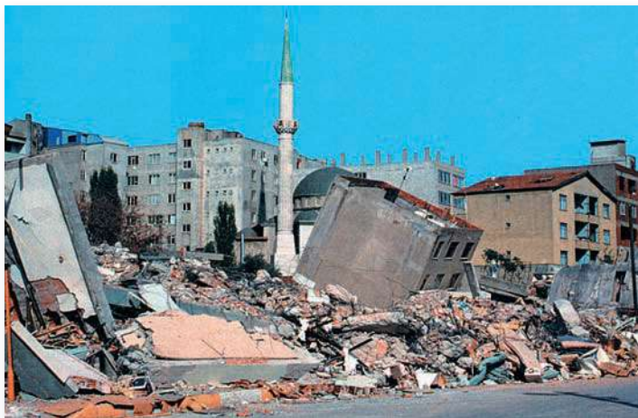
FIGURE 14.17 An earthquake near the town of Izmit in western Turkey in 1999 killed at least 50,000 people and injured an equal number. Poorly constructed buildings collapsed and trapped residents, while stronger structures nearby remained standing.
