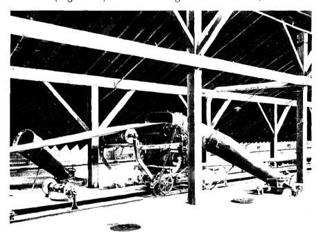
Figure 9–2. The movable automatic "dump" takes grain from the belt conveyor and spouts it into the top of a bin.
