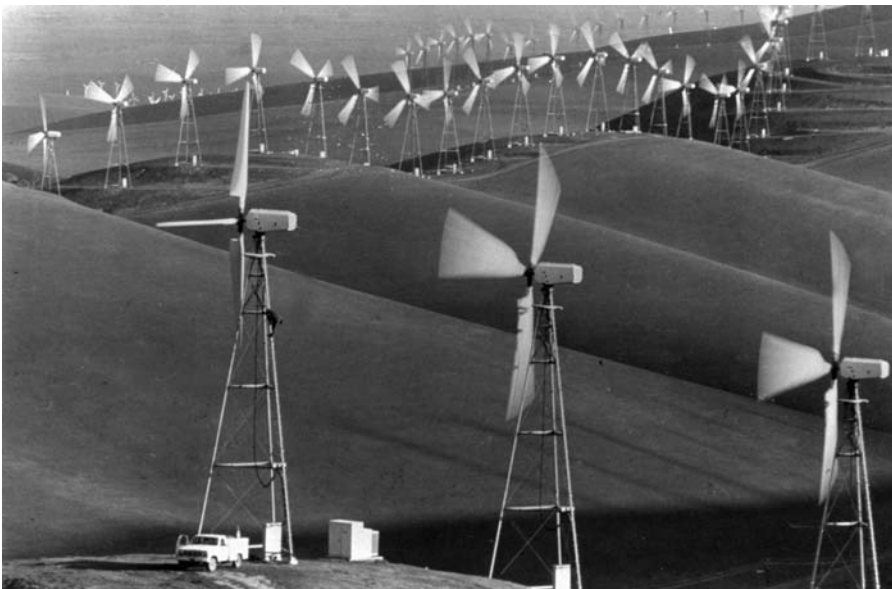
Figure 183 A wind-powered electrical generation station near Livermore, California.
