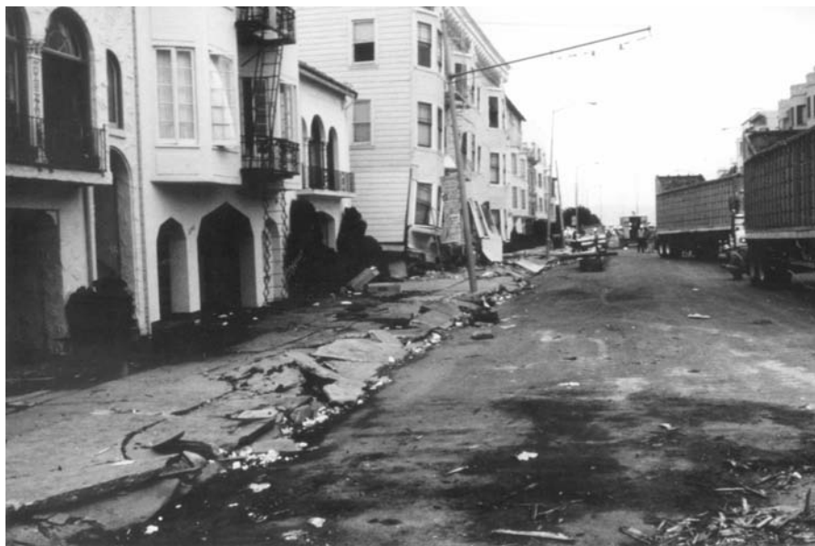
Figure 102 Buildings damaged in the Marina district, San Francisco from the October 17, 1989, Loma Prieta, California, earthquake.
