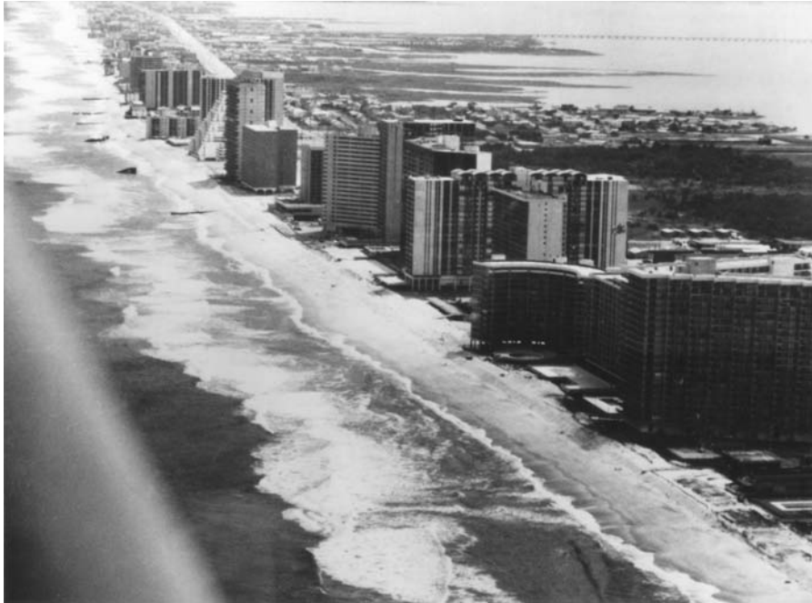
Figure 75 Development along the shoreline Ocean City, Maryland. The distances between these buildings and the shoreline leave little room for natural processes during storms.
