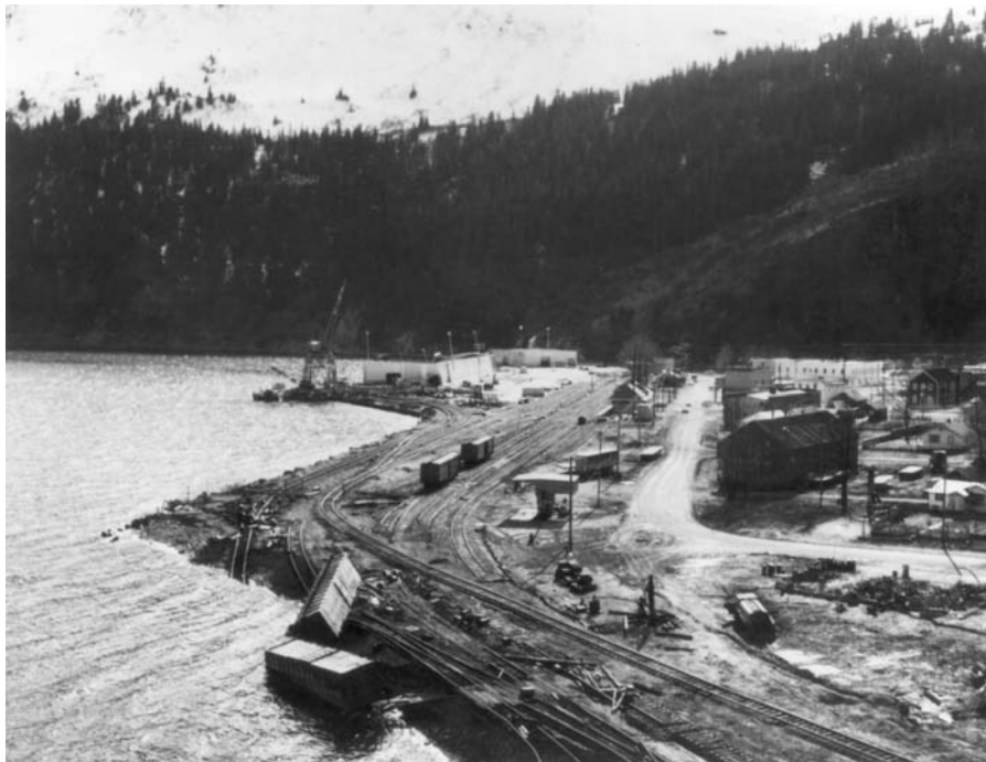
Figure 133 A railroad yard and warehouse damaged at Seward due to submarine slides from the March 27, 1964, Alaskan earthquake.
