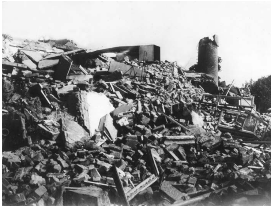
Figure 199 Rubble from a brick building that completely collapsed during the July 28, 1976, Tangshan, China, earthquake that killed 250,000 people.
