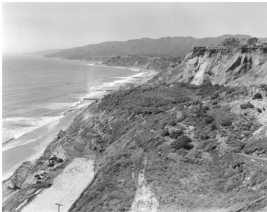
Figure 128 A landslide that extends over the Pacific Coast Highway, the Pacific Palisades areas, Los Angeles County, California, on March 31, 1958.
