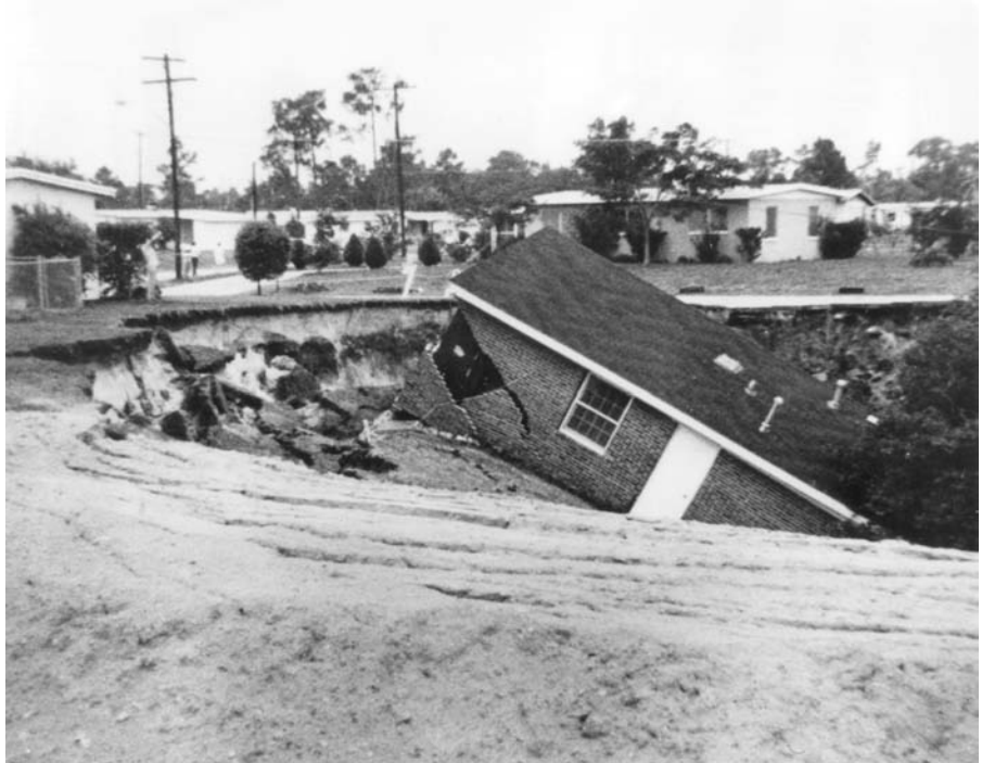
Figure 142 A sinkhole 520 feet long, 125 feet wide, and 60 feet deep that collapsed under a house in Barton, Florida.
