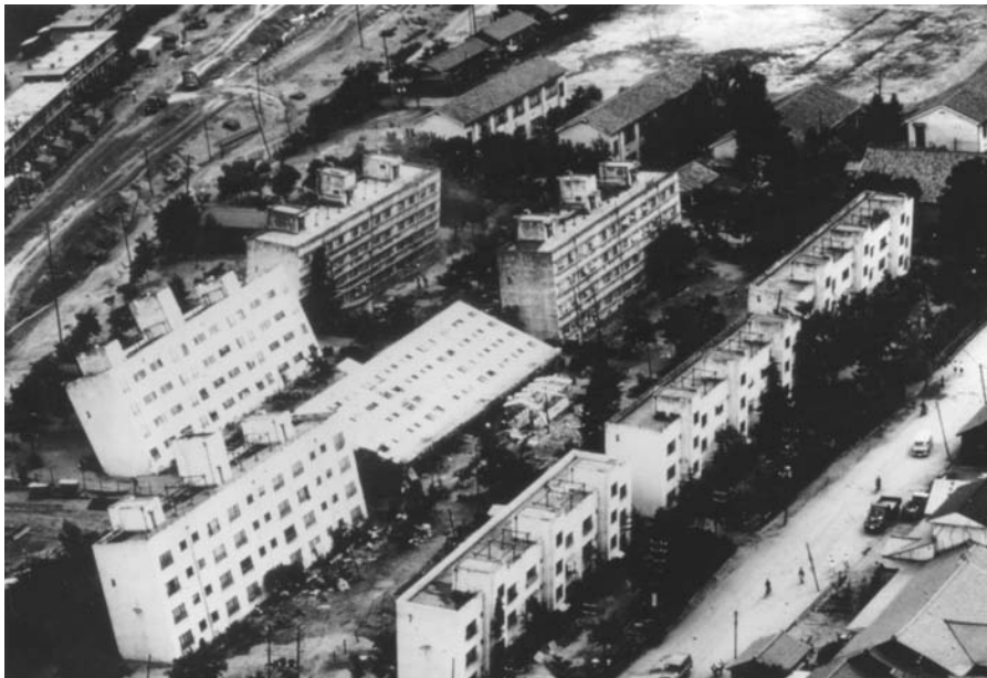
Figure 138 Apartment buildings in Niigata, Japan, that tipped because of the loss of bearing strength caused by liquefaction in the underlying sediments during the 1964 Niigata earthquake.
