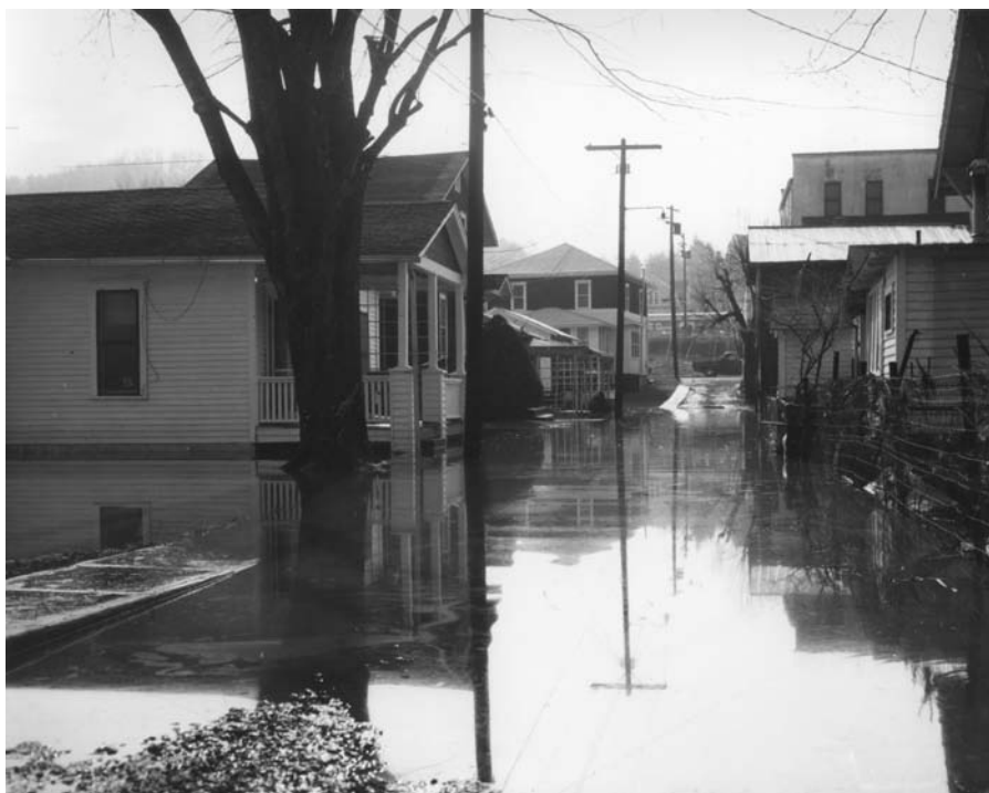
Figure 201 Damage to homes in Grantsville, West Virginia, caused by flooding of the Little Kanawha River on March 6, 1967.
