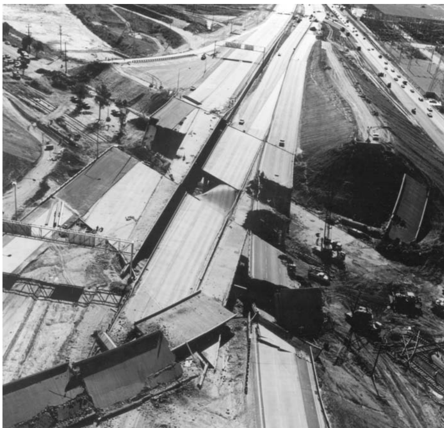
Figure 99 Collapsed freeway overpass from the February 9, 1971, San Fernando, California, earthquake.
