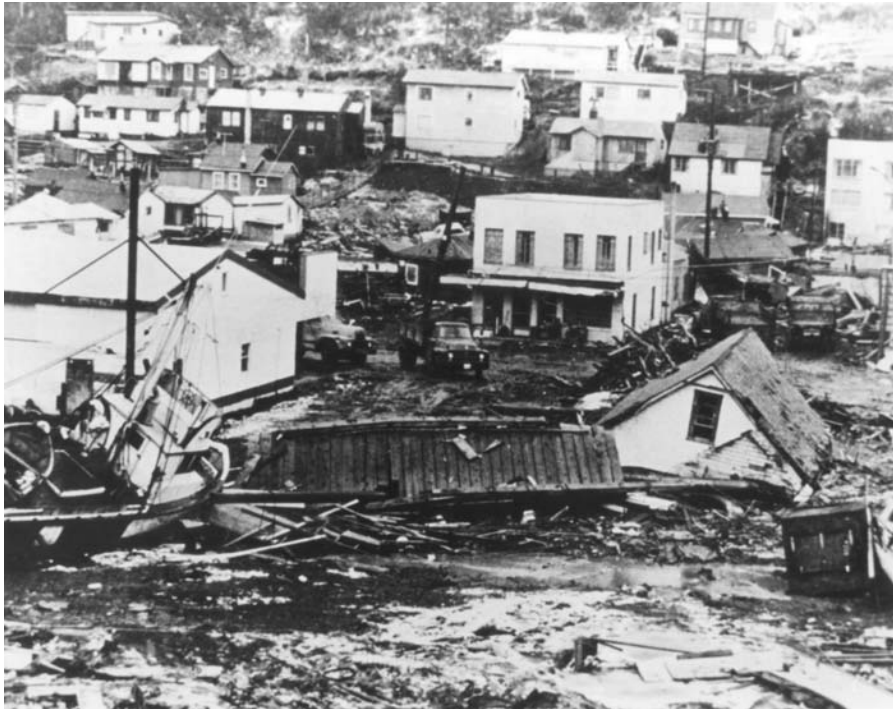
Figure 93 Tsunamis destruction of Kodiak Island from the March 27, 1964, Alaska earthquake.
