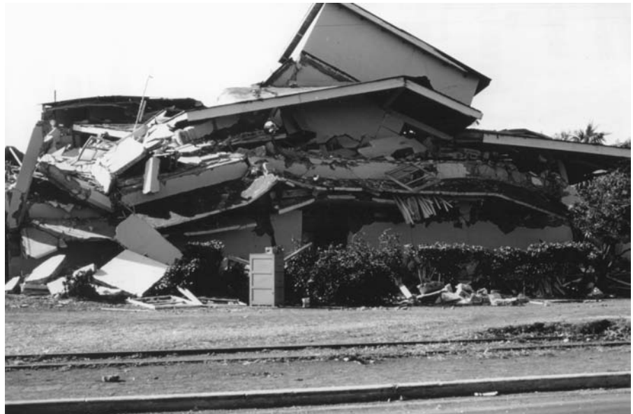
Figure 100 A collapsed three-story Customs House office building, from the December 23, 1972, Managua, Nicaragua, earthquake.
