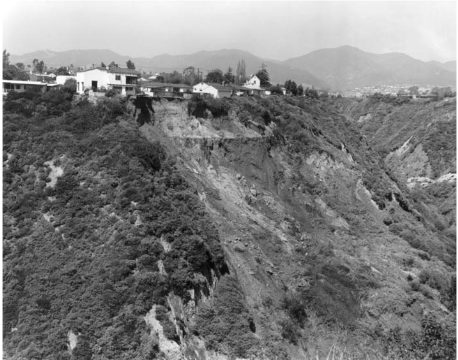
Figure 129 Slumping of unstable earth materials undermines the foundations of houses in the Pacific Palisades area of southern California.
