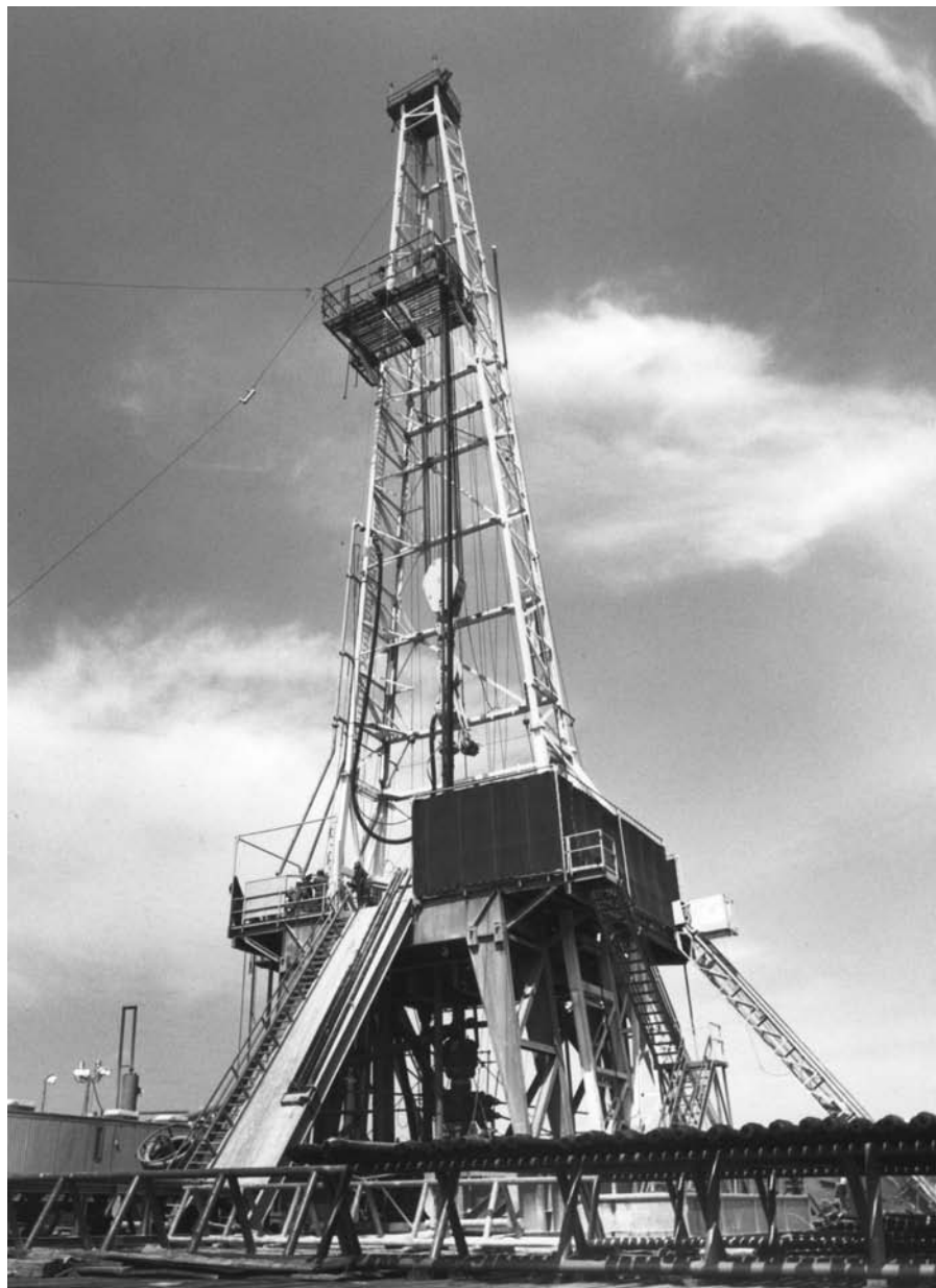
Figure 168 A drilling rig used to extract geopressed energy near Houston, Texas.
