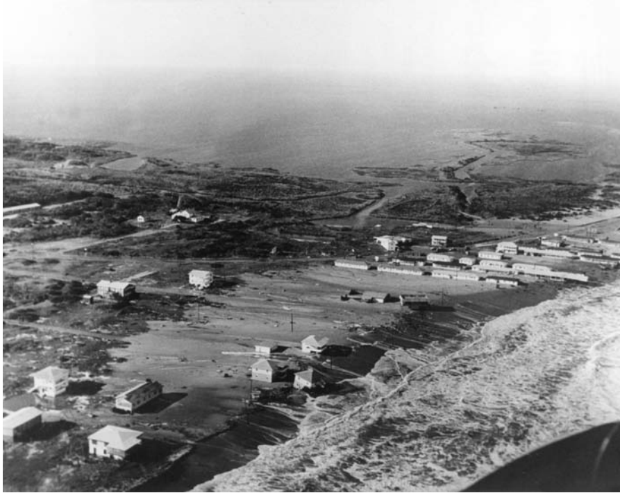
Figure 91 Overwash and storm surge penetration near Cape Hatteras, North Carolina, in 1962.
