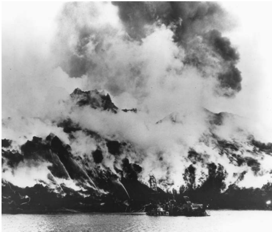
Figure 117 Seawater is being sprayed directly onto a lava flow in the outer harbor of Vestmannaeyjar, Iceland, from the May 4, 1973, eruption on Heimaey to arrest it from infilling the harbor entrance.
