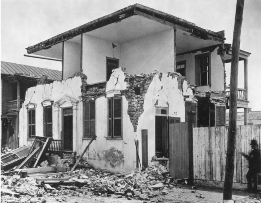
Figure 98 Wreckage from the August 31, 1886, Charleston, South Carolina, earthquake.
