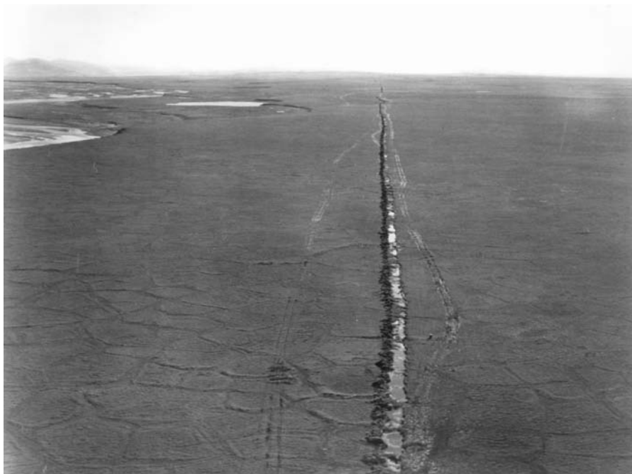
Figure 190 Tractor trail on the North Slope of Alaska. The small ponds are due to thawing of the permafrost in the roadway.
