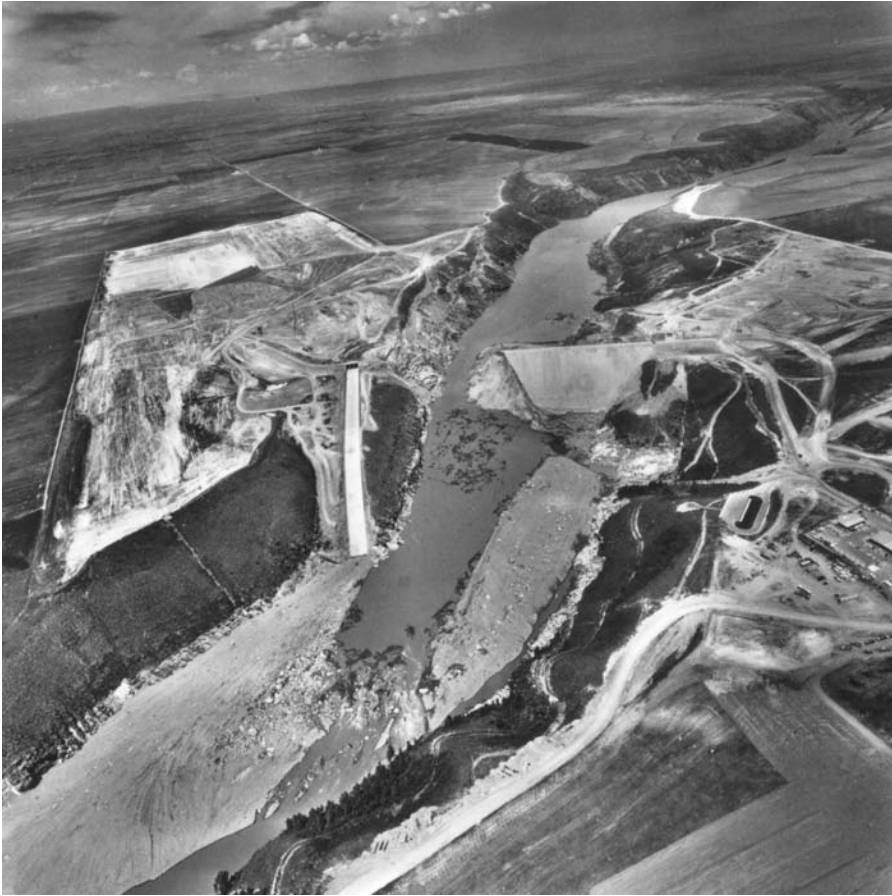
Figure 71 The June 5, 1976, Teton Dam break, which caused extensive flooding downstream.
