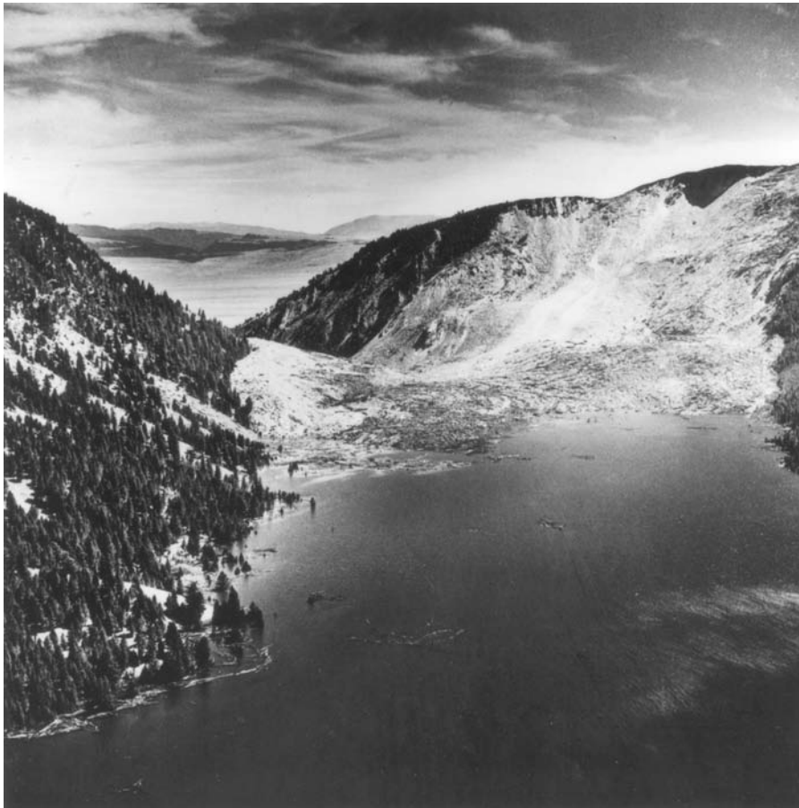
Figure 130 The August 1959 Madison Canyon slide, Madison County, Montana.
